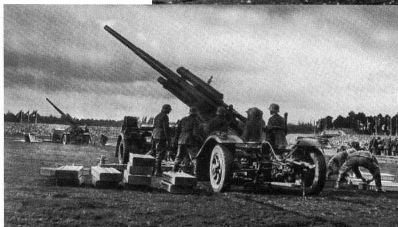
LEFT: The superb 8.8cm Flak that would prove as effective as an anti-tank gun as it was an AA gun. During the war new carriages would be developed to give it a lower silhouette.
