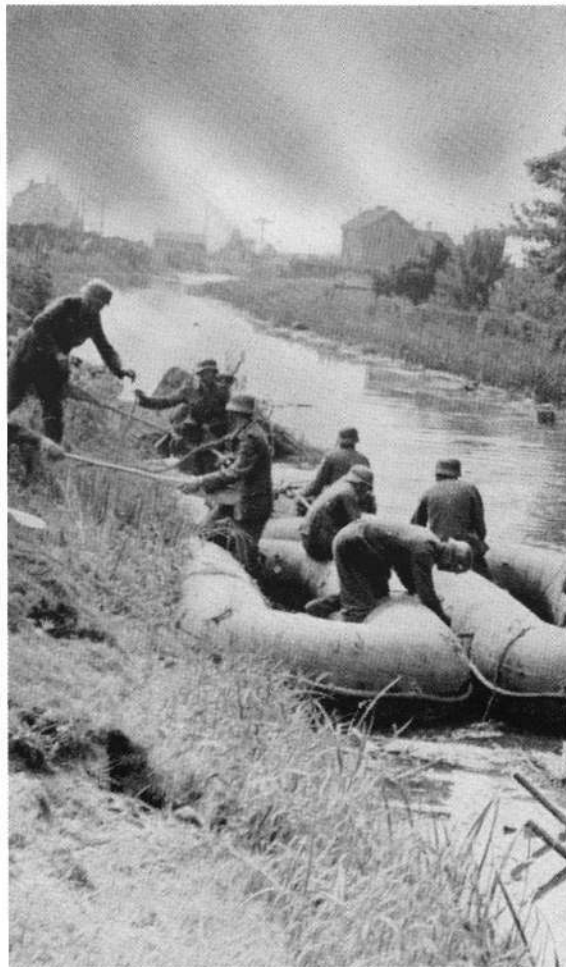
ABOVE: Medium Pneumatic Boats are linked into an assault bridge across a canal in France by German Pioniere . The boats were 5.5m (18ft) long and weighed 150kg (330lb) and could carry seven men.
