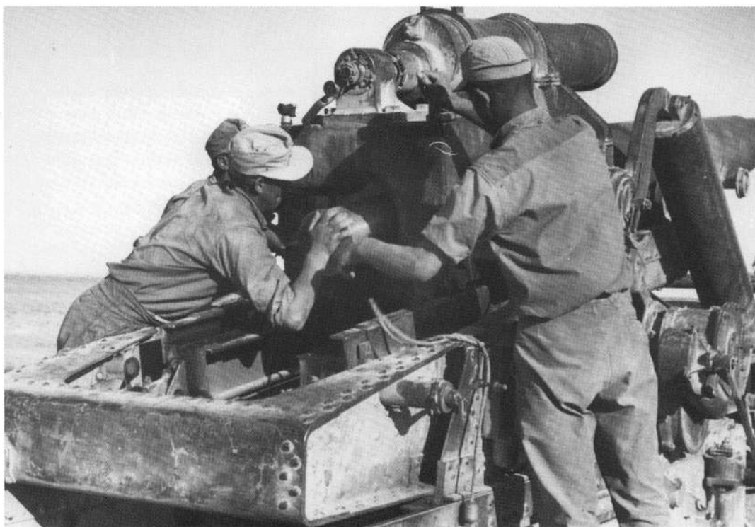
ABOVE: Afrika Korps gunners load a 21cm Mörser 18 howitzer. The big gun could fire one 133kg round every two minutes.
