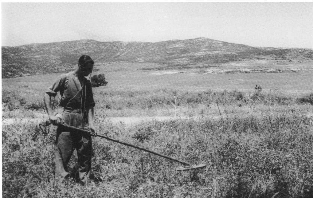
ABOVE: A British sapper uses an electronic mine detector to locate mines near the Medjez-Tebourba road, Longstop Hill, Tunisia in April 1943.
