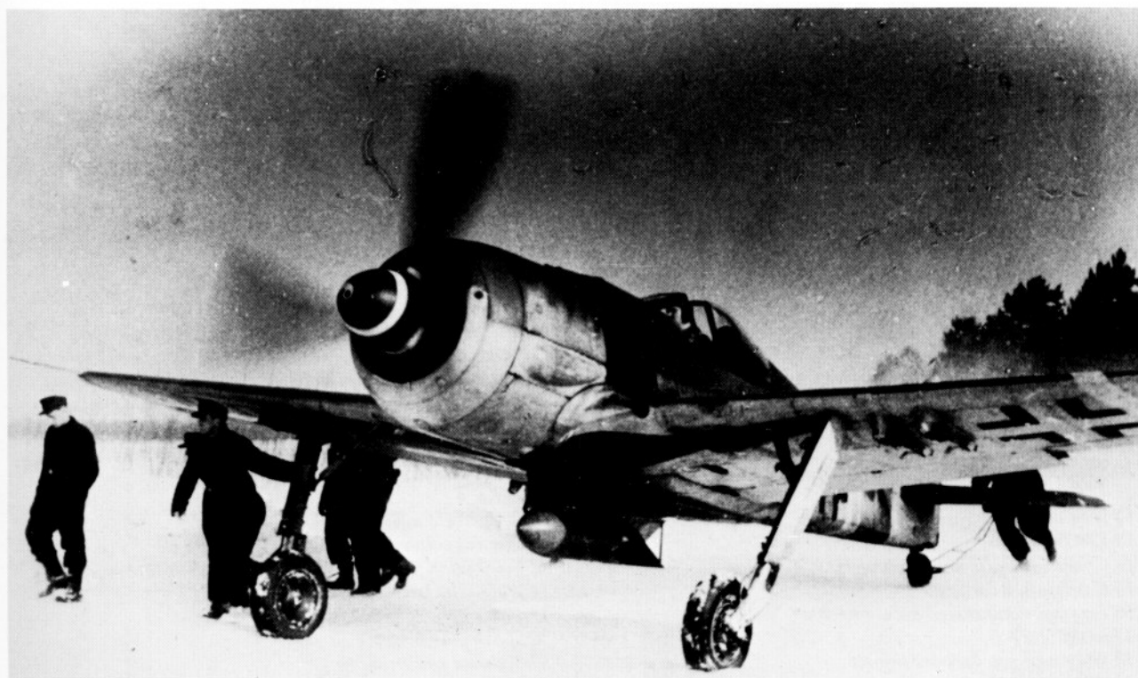
Fw 190F-8/R1 with four ETC 50 bomb racks beneath the wings and an ETC 250 rack under the fuselage, occupied by a 250-kg bomb.
