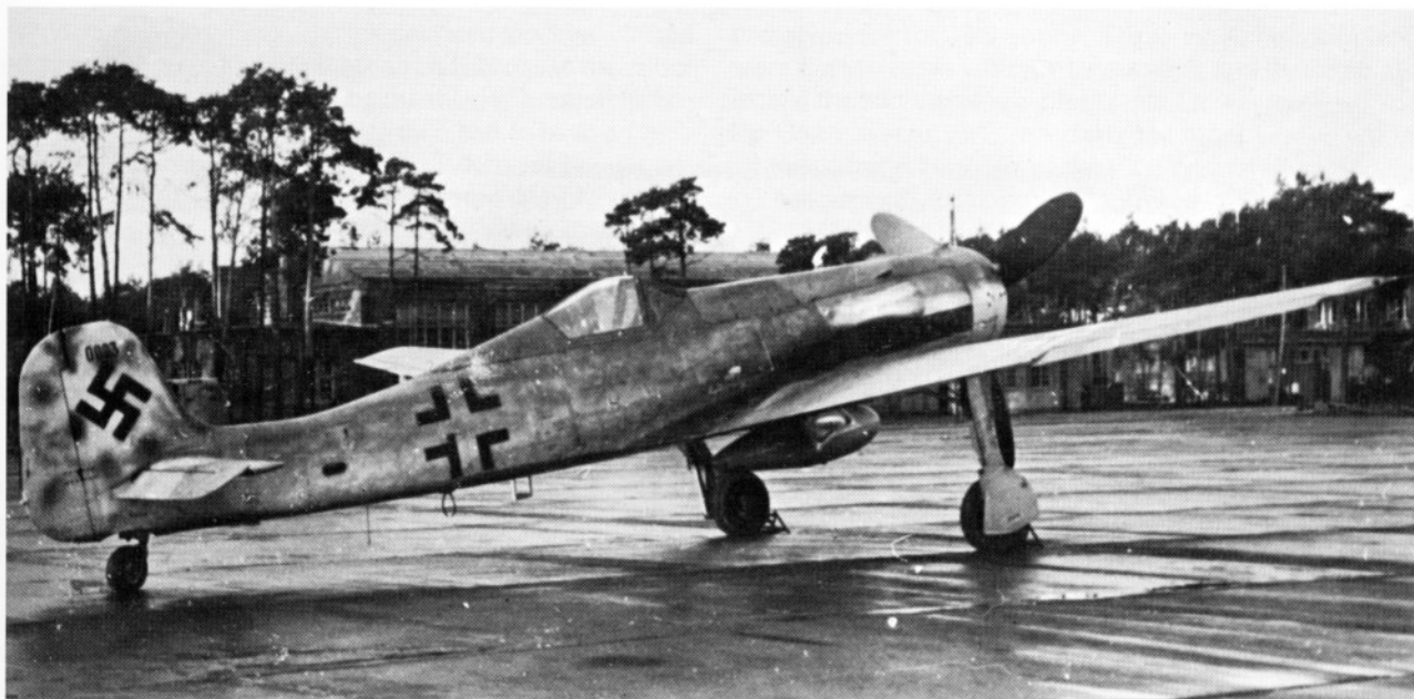
Ta 152H-0 (Werknummer 150003) with Jumo 213E at the Langenhagen factory, 1945.
