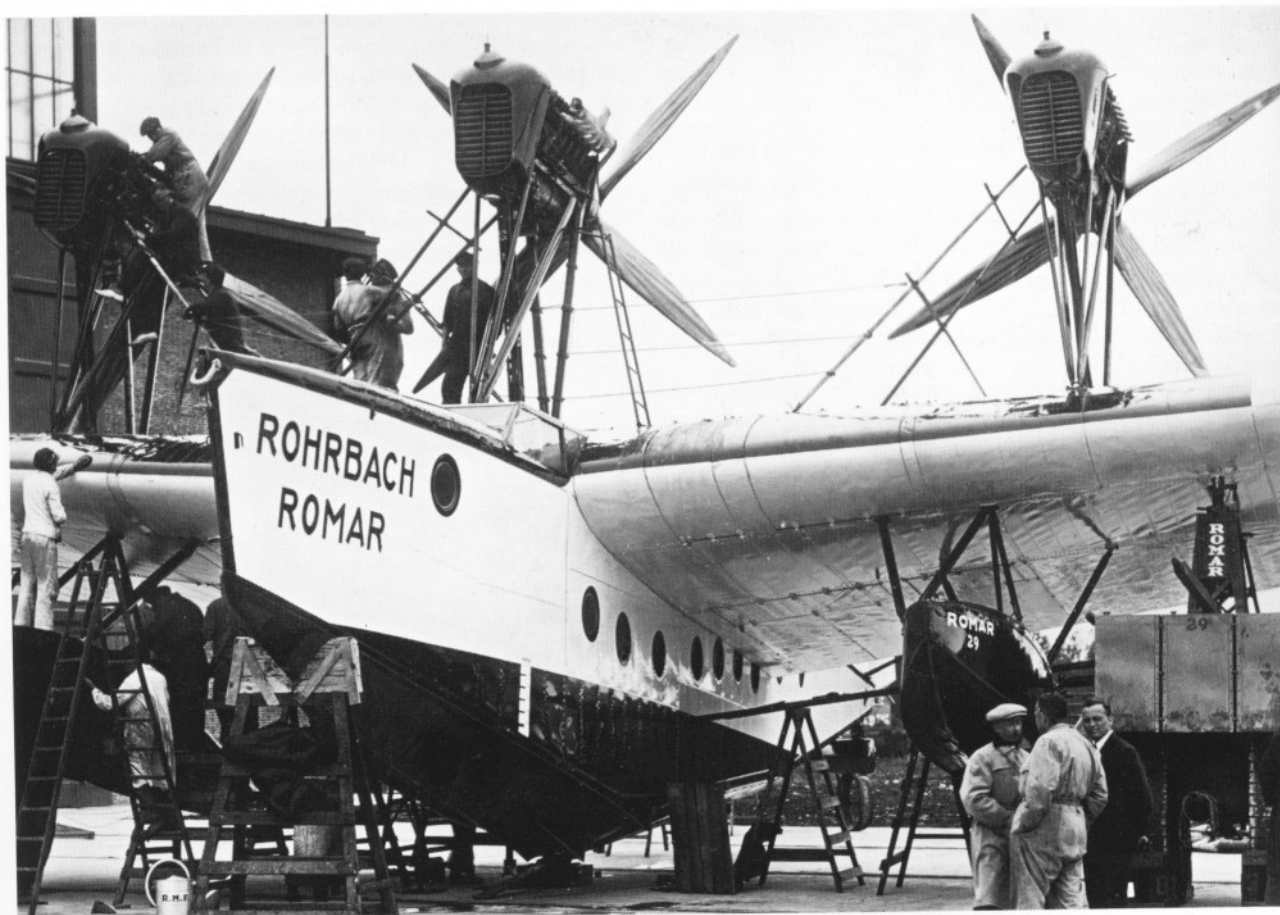
Rohrbach Ro X Romar I with three BMW VI engines having front radiators and four-bladed propellers (Werknummer 29).
