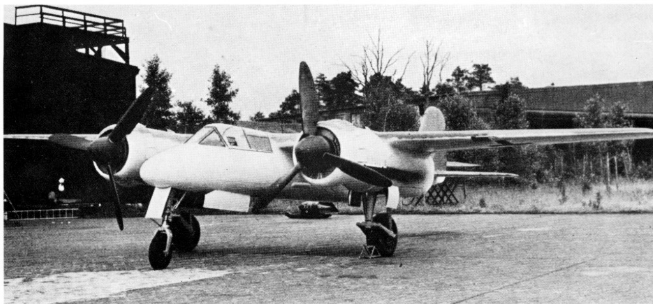
Ta 154 V1 TE+FE with Jumo 211 F/2 in July 1943 at Hannover-Langenhagen.
