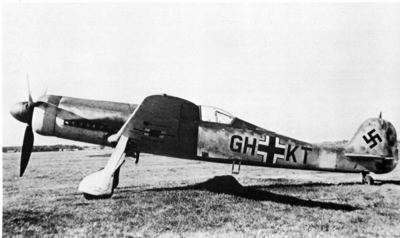
An Fw 190 V30/U1 (0055) with Jumo 213E, modified to Ta 152H-0 GH-KT. Photo taken on 8/13/1944.
