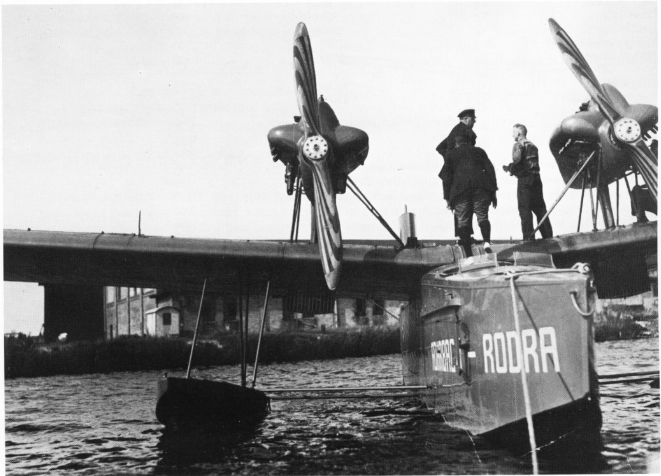
The Rohrbach Ro IIIa Rodra with two Lorraine Dietrich engines, each having an output of 330 kW (450 hp). Two of these flying boats were delivered to Turkey in 1926.
