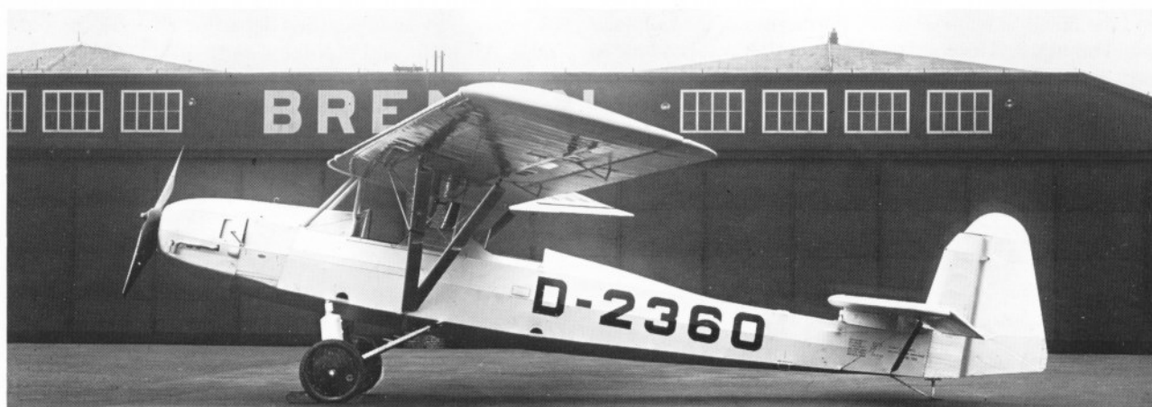
AL 103 experimental and research aircraft with wings which could be adjusted in their dihedral and sweep.
